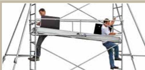
**INSTALLATION EN SÉCURITÉ DU PLANCHER**
